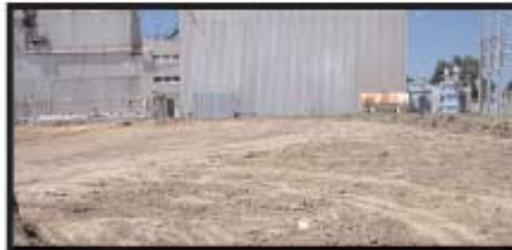
Site Preparation August 7th, 2009
